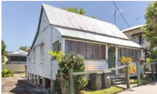
21 Clay Street, New Farm
