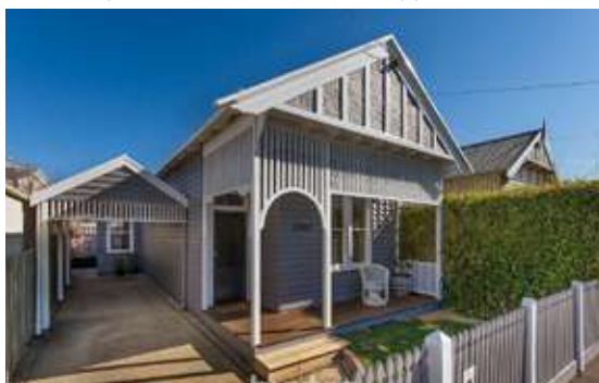
22 Walker Street, Ripplside
